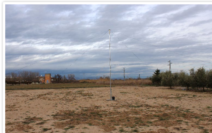
Fig. 14: Beacon transmitter 6 installed on a vacant building site in Menarguens.
